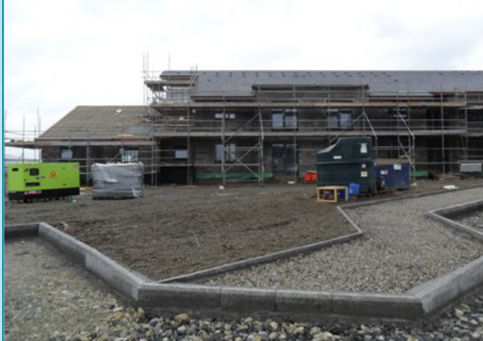
Mull Progressive Care Centre under construction
